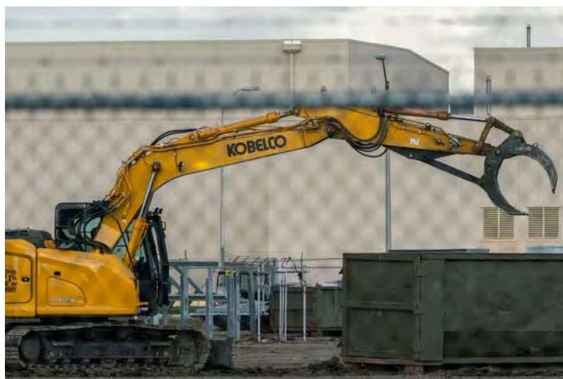
A data center under construction last October in Lordstown, Ohio. KYLE GRILLOT/BLOOMBERG NEWS
