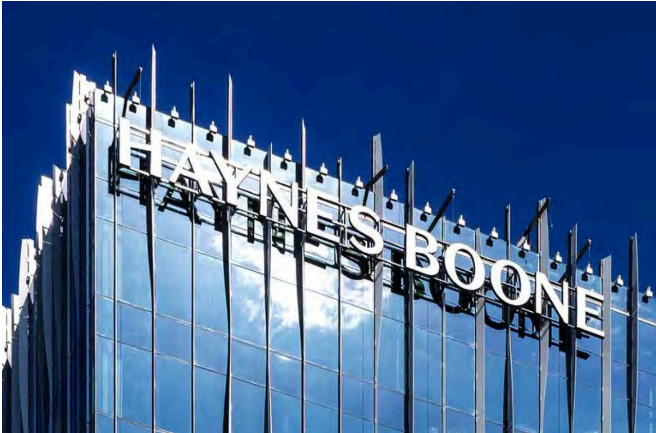
Haynes and Boone offices in Dallas, TX. Courtesy photo
