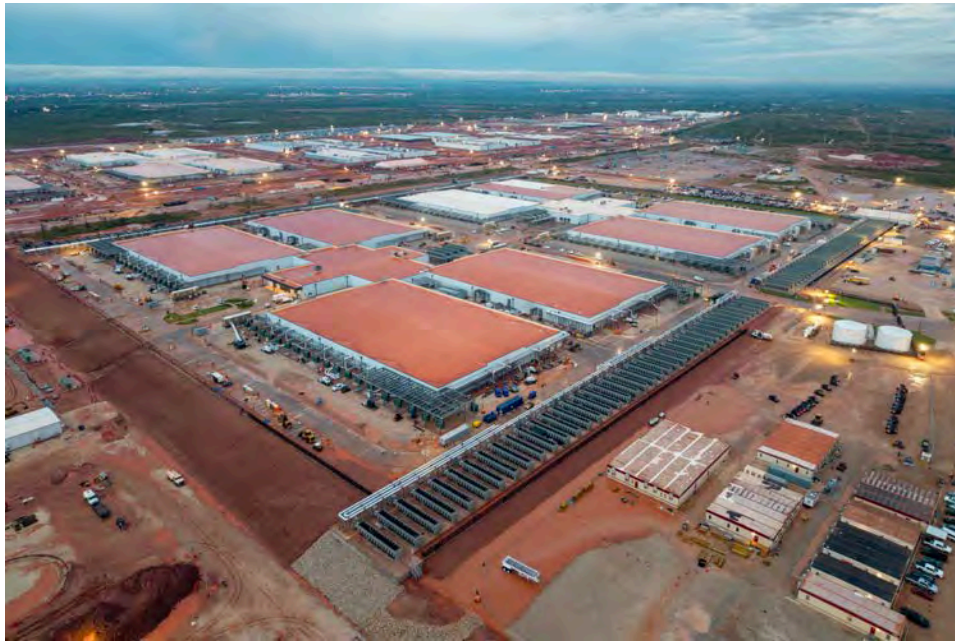
Construction of the first Stargate AI data center, in Abilene, Texas.
