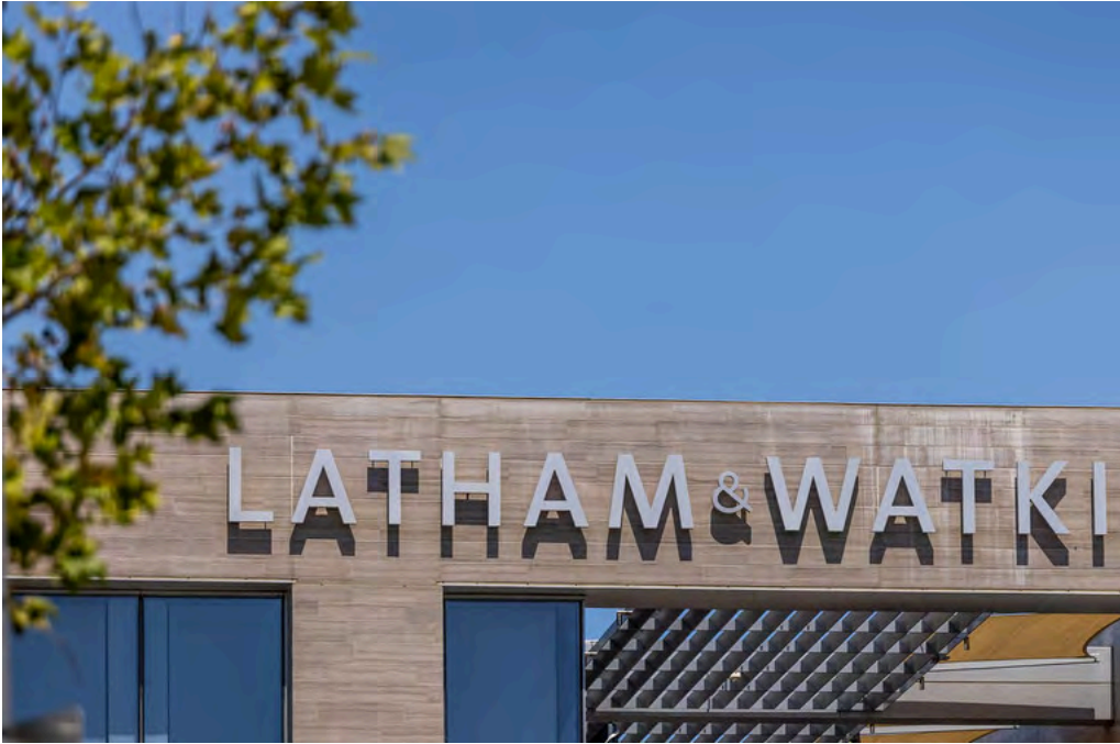
Latham & Watkins offices in San Diego, CA. Photo: Jason Doiy
