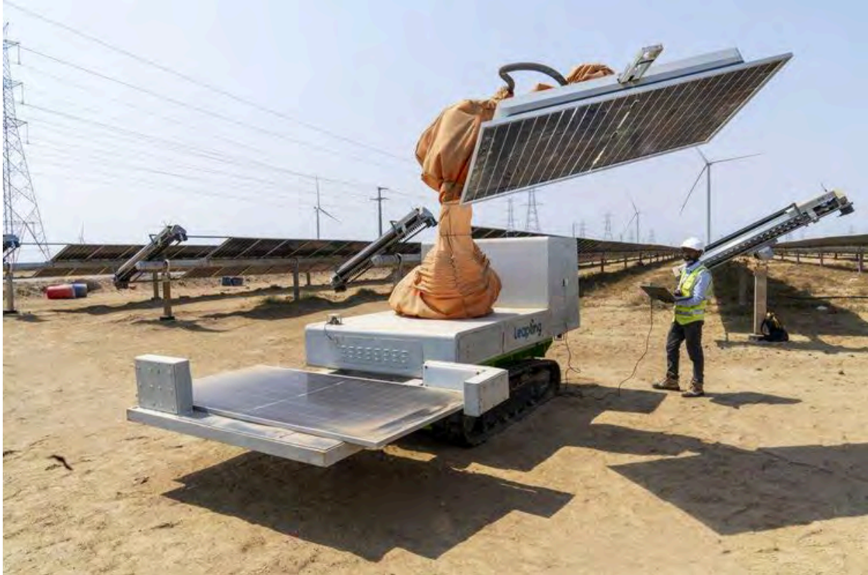
Installation of solar panels at Adani Green Energy's Khavda Renewable Park in Gujarat in May.
