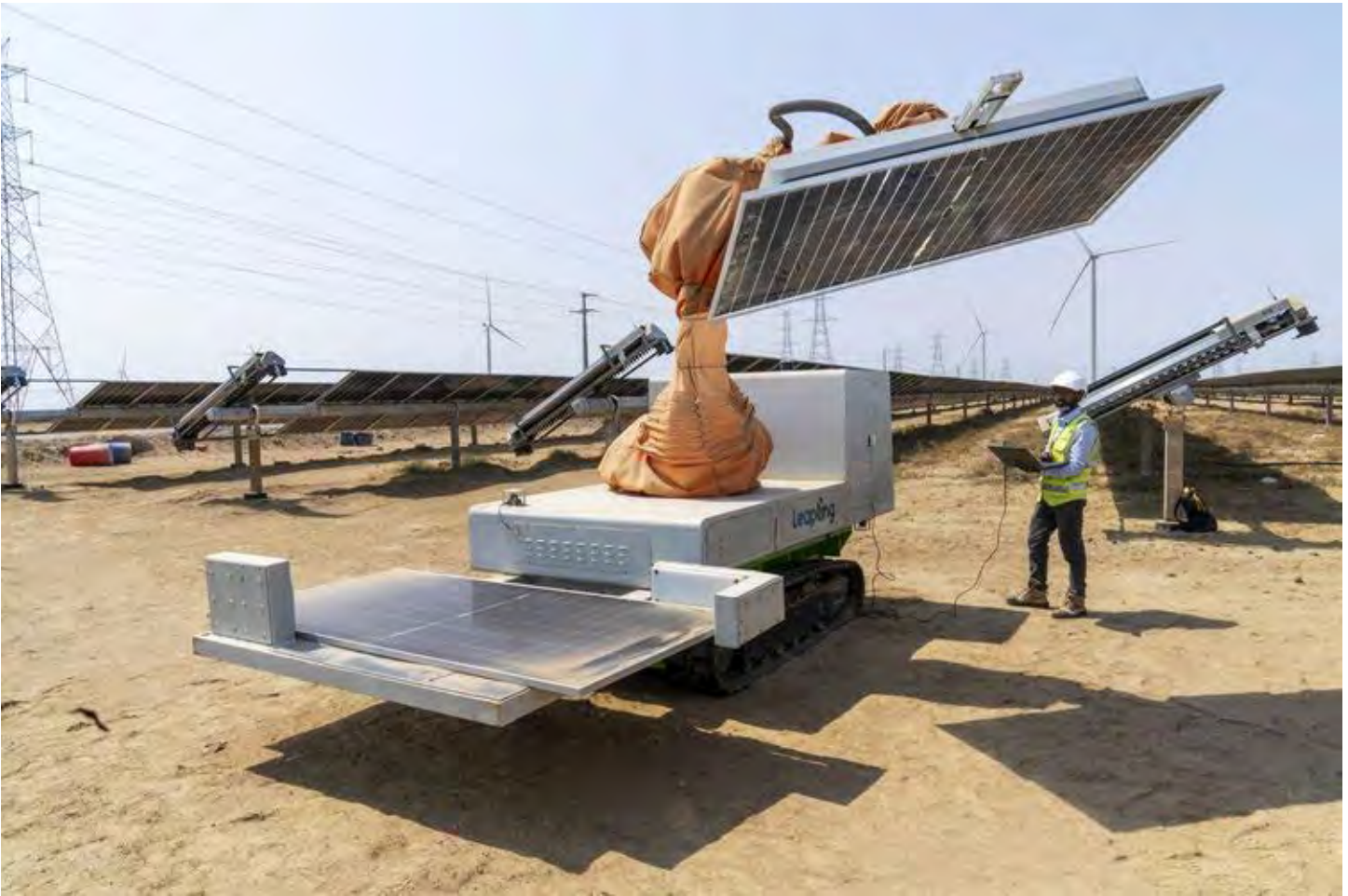
Installation of solar panels at Adani Green Energy's Khavda Renewable Park in Gujarat in May. Photographer: Sumit Dayal/Bloomberg
