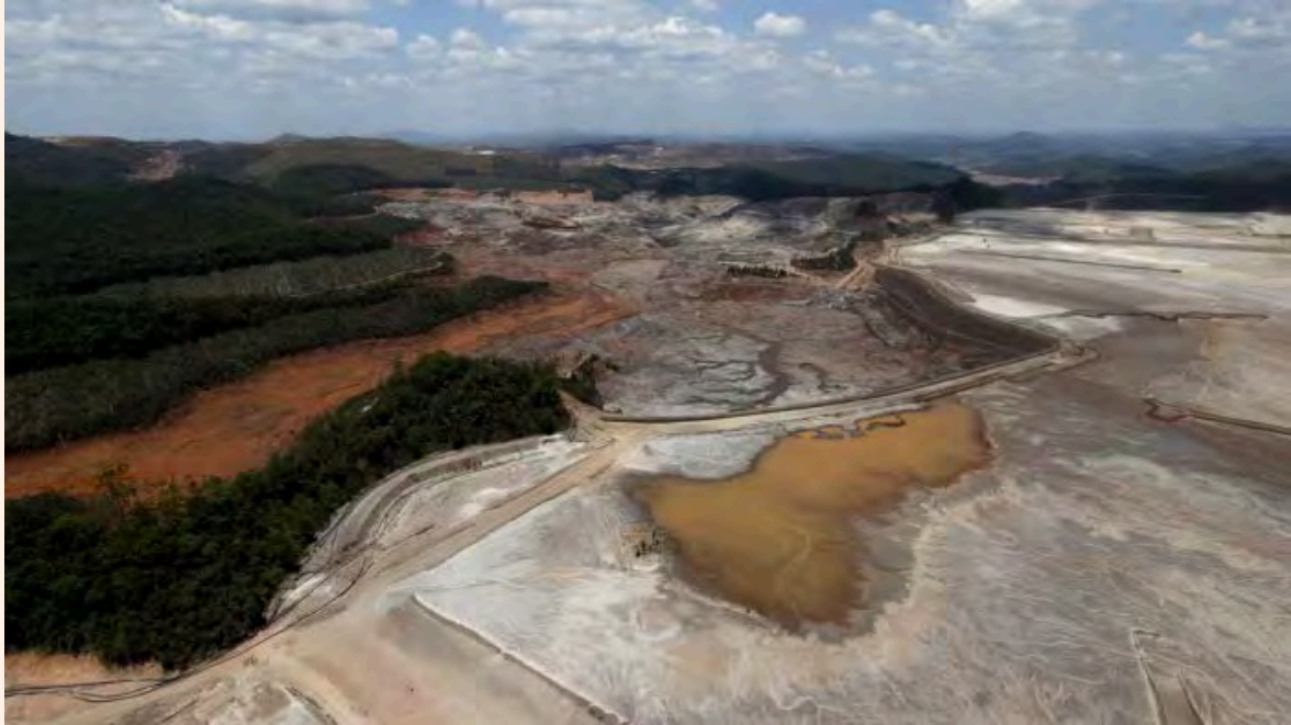
An aerial view of the dam owned by Vale and BHP after it burst in Mariana, Brazil, in 2015 © Ricardo Moraes/Reuters
