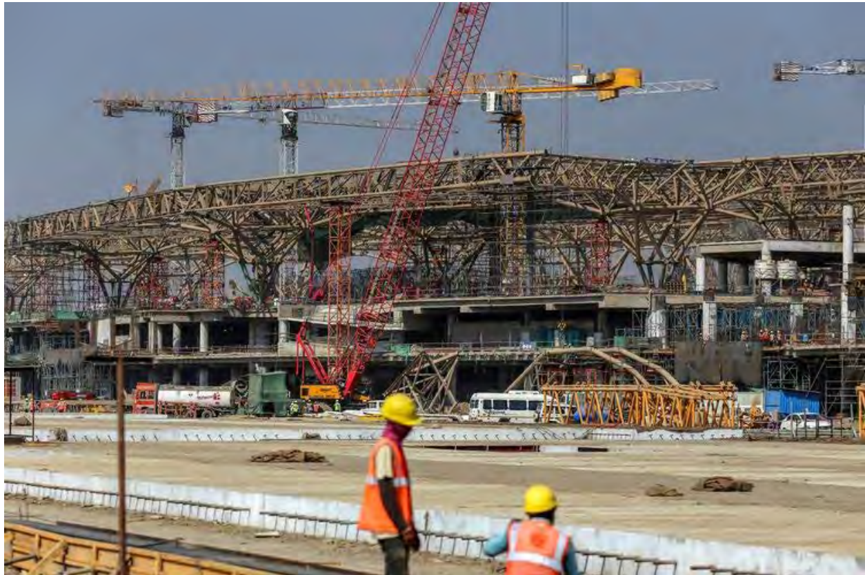
A building under construction at the Navi Mumbai International Airport in Navi Mumbai, India, on Feb. 23, 2024.
